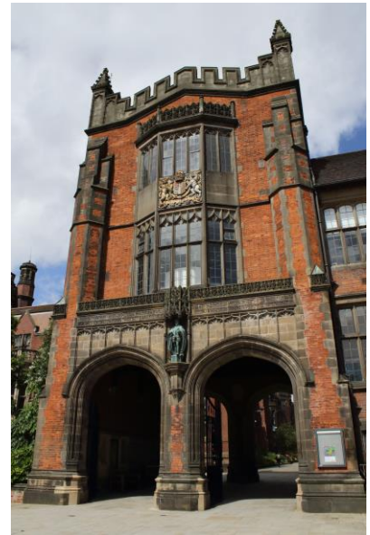
Photo on right: ‘The Arches’ of Armstrong Building, Newcastle University, 28 July 2017.
