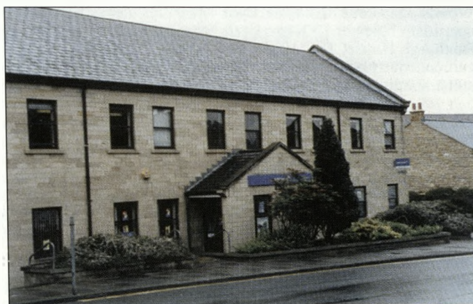
Fig. 12 Roxburgh House (ca 1970) in Green Batt, Alnwick built of Coal Measures sandstone probably from near Bradford.
