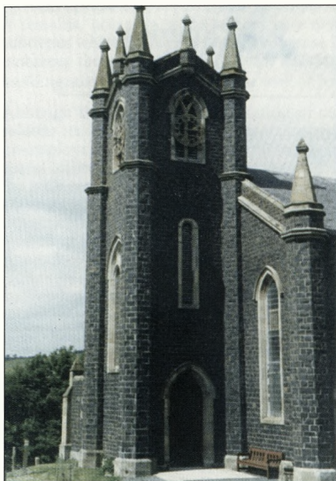
Fig. 2 Yetholm Church (1836) with walls of dressed black basalt and doors and windows of dressed sandstone.
