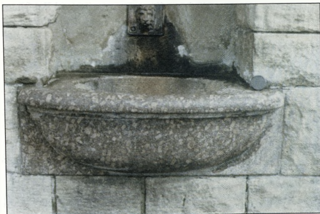
Fig. 13 Shap Granite basin on the Denton Memorial Fountain, Alnmouth designed by G. Reavell and built in 1924-25 by J. G. Green of Warkworth for a cost of £299. Note the large crystals of orthoclase feldspar.
