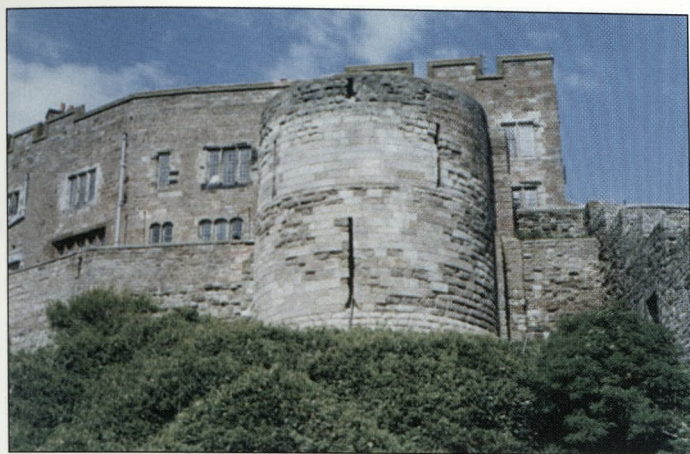
Fig. 6 West end of Bamburgh Castle rebuilt in the early 1900s using Penrith Sandstone from Lazonby.
