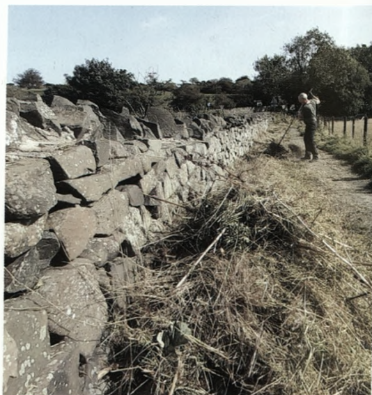
Dry stone wall repair. Image © Em Witcutt.
