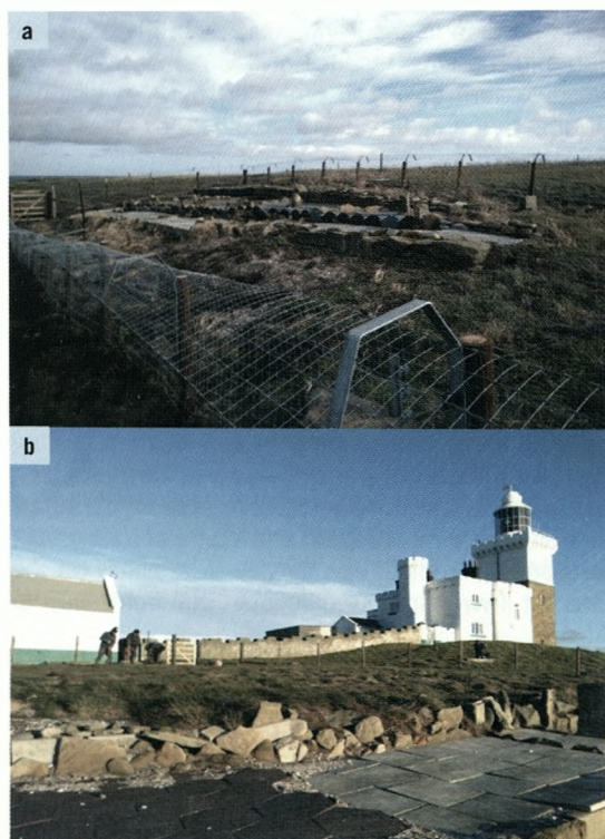
Figure 1. The north terrace fence (a) and the south terrace (b) under construction.
