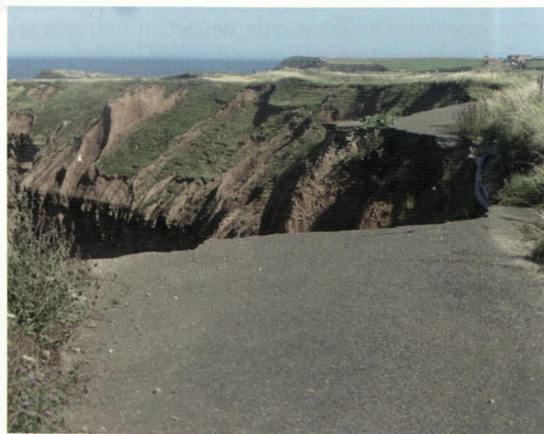
Figure 8. Coastal erosion in superficial (drift) geological deposits at Cowbar in Redcar & Cleveland.
